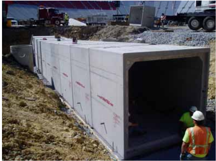
Precast concrete pedestrian tunnel and site utilities at BMS.
